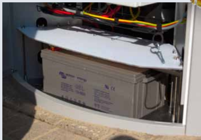
Photo 6 & 7: The Victron batteries and the MultiPlus are fitted in the pillar.
