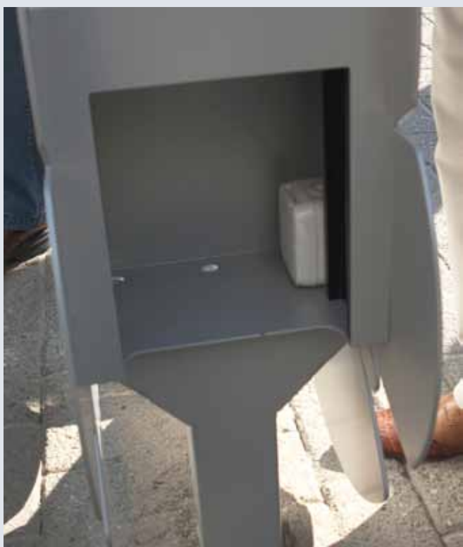
Photo 8 & 9: The charge point is surrounded by a waterproof enclosure, which can be shoved upwards.
