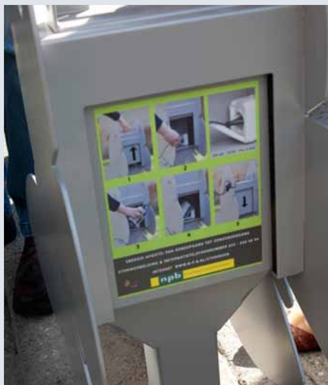
Photo 8 & 9: The charge point is surrounded by a waterproof enclosure, which can be shoved upwards.
